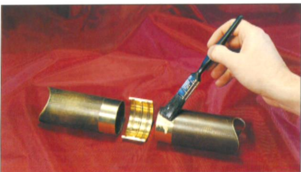
G - Add flux to tube and fitting
